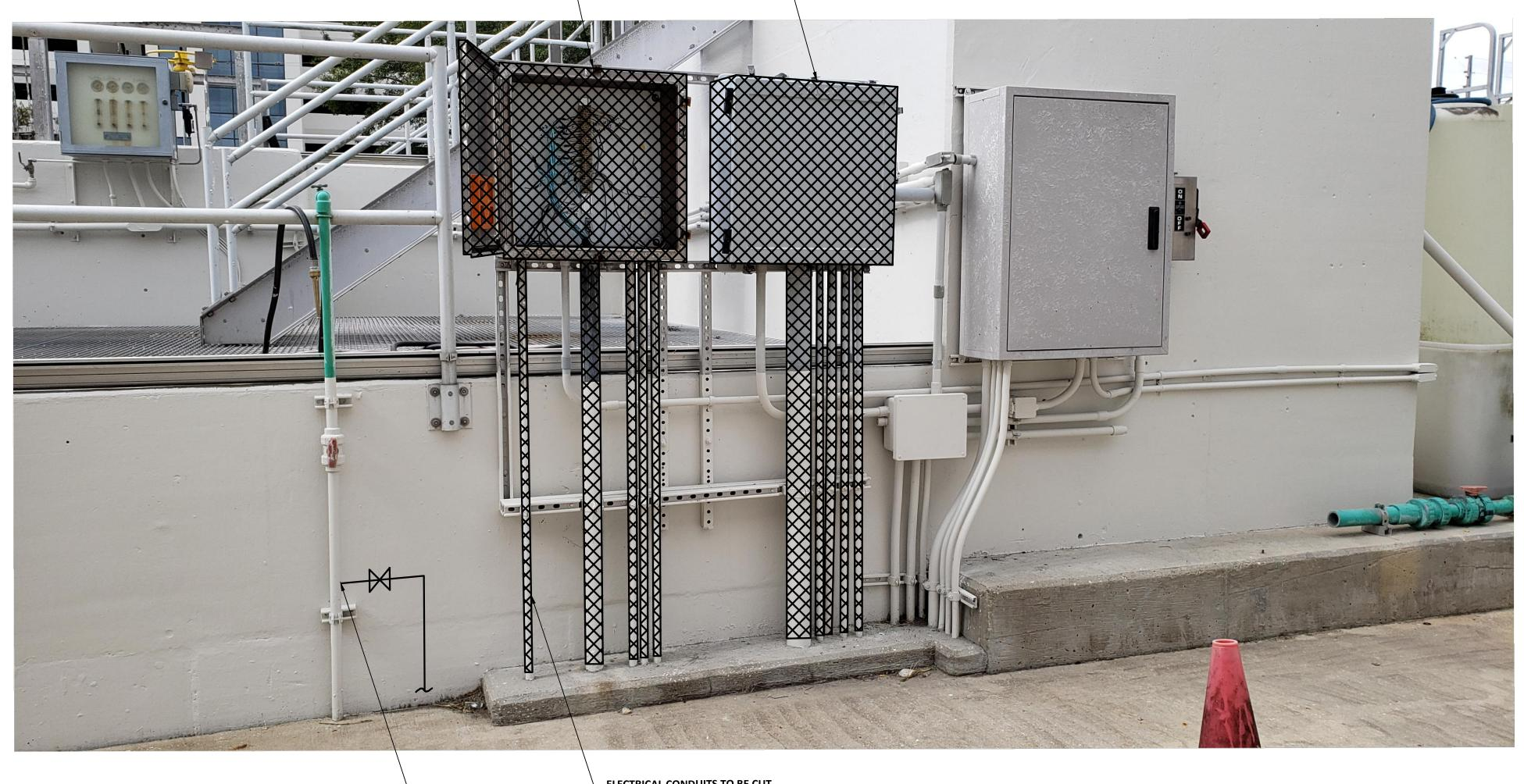
ELECTRICAL CONDUITS TO BE CUT AND CAPPED AT GRADE (TYP.)
