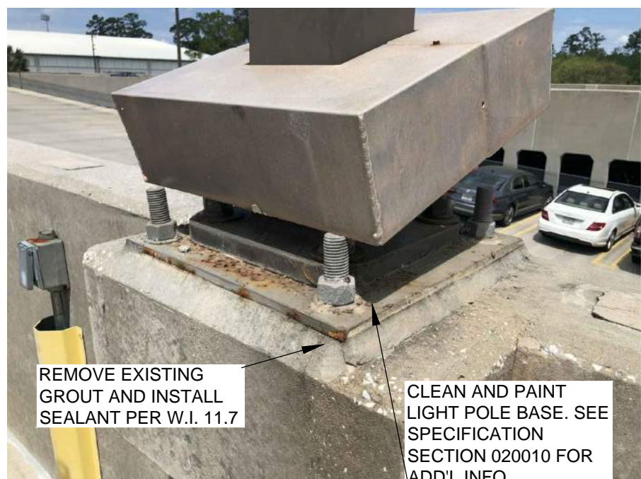
45.8 CLEAN AND PAINT LIGHT POLE BASE
