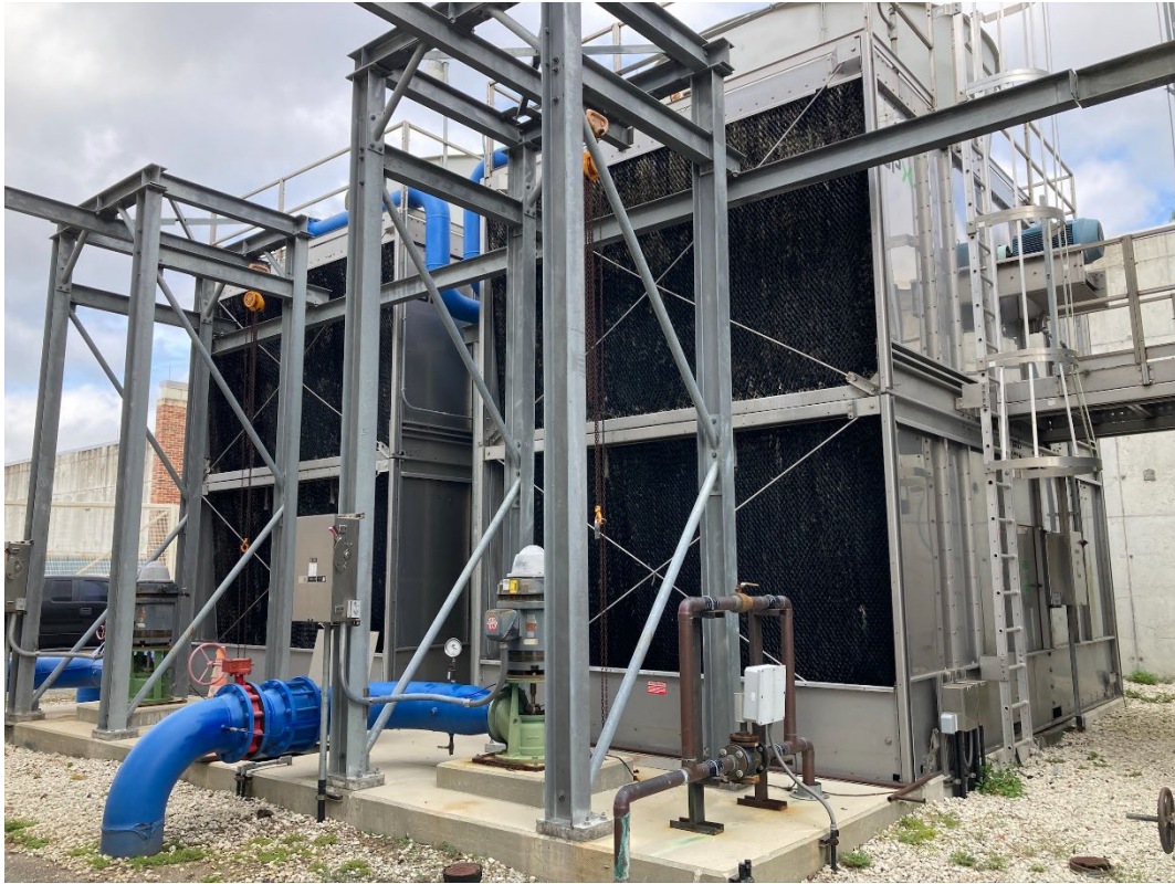
Cooling Towers 3 & 4 Looking SE to NW (Pump Side of Towers – “Front”)
