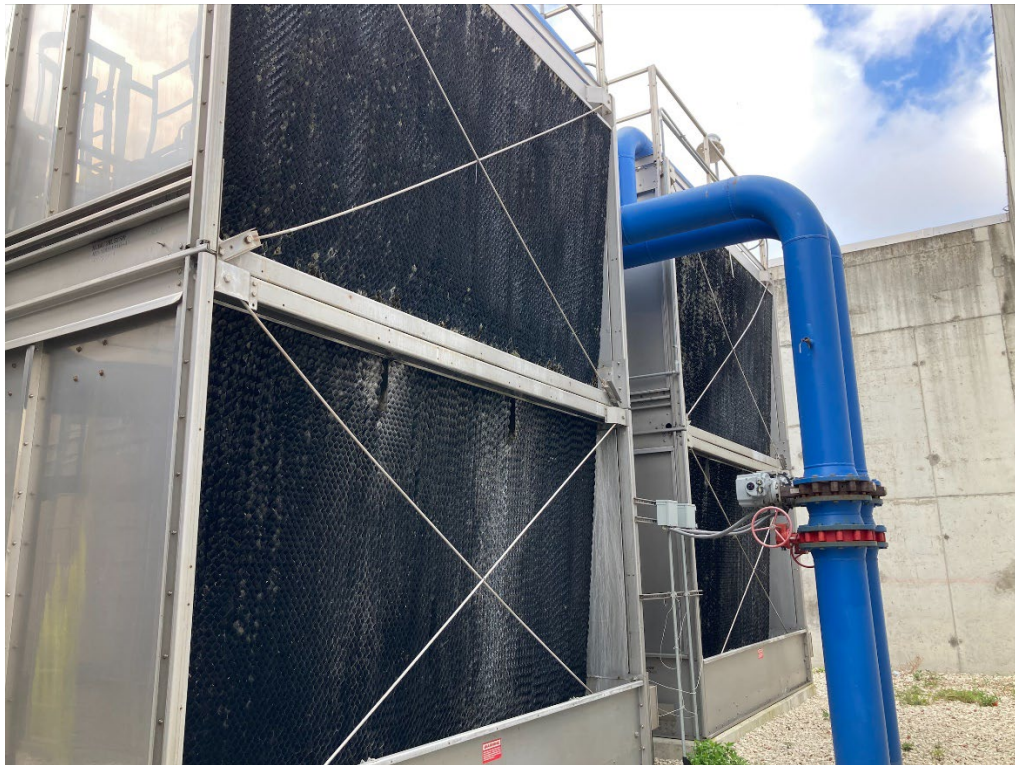
Cooling Towers 3 & 4 Looking NE to SW – (“Rear” of Cooling Towers)
