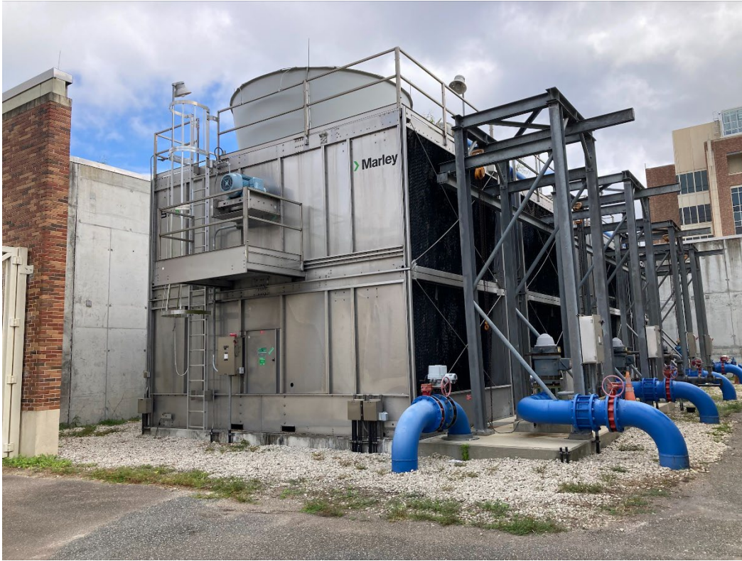
Cooling Towers 3 and 4 Looking from the SW to NE
