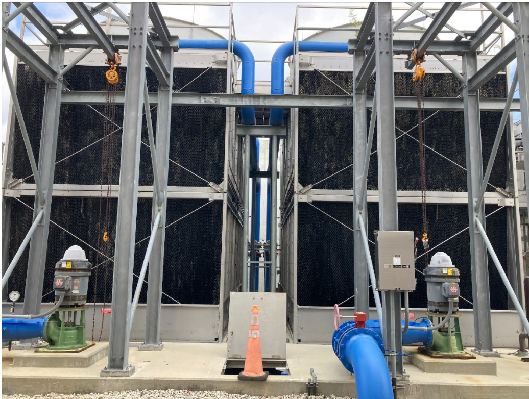
Cooling Towers looking From South to North (Pump Side of Towers – “Front”)
